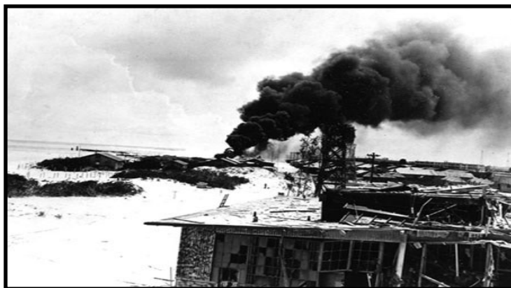
Japanese carrier-launched bombers have withdrawn after striking Midway on the morning of 4 June 1942. In this view of Sand island, the camera is facing south-west and shows the bomb-damaged laundry building in the foreground and burning oil tanks in the distance. Ed Fox's machine-gun bunker was located beyond the burning oil tanks and on the shore line
